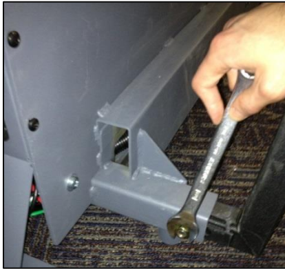
Figure 29 - Attach Caster to Frame
