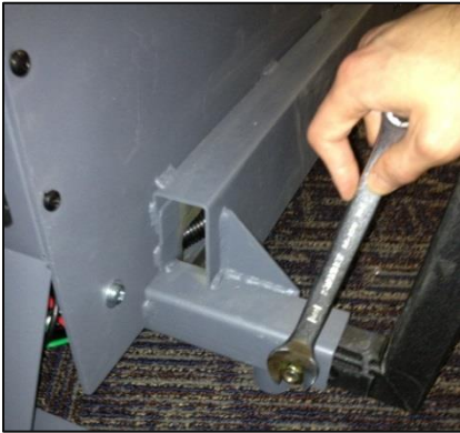
Figure 29 - Attach Caster to Frame
