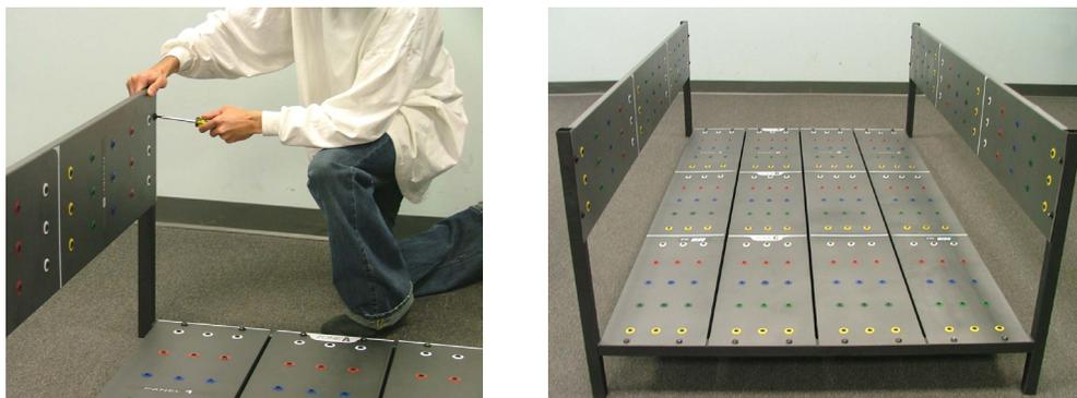
Figure 1-11. Attaching FROM Panel 6 and Completed Assembly
